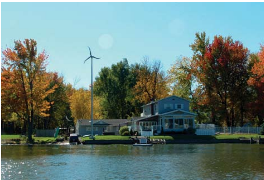
Wide open spaces generally provide the best wind conditions, as obstructions cause the wind to slow.
