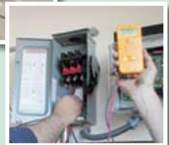
Below: Testing PV array voltage.
